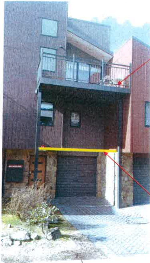
Existing deck structure
